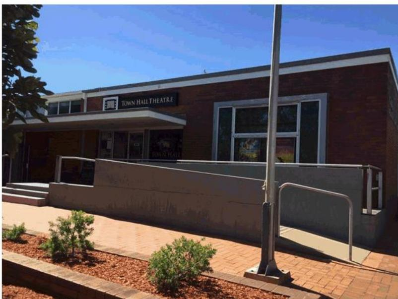
**Photo 9: Existing ramp to be modified during construction. Existing flagpole to be removed.**
