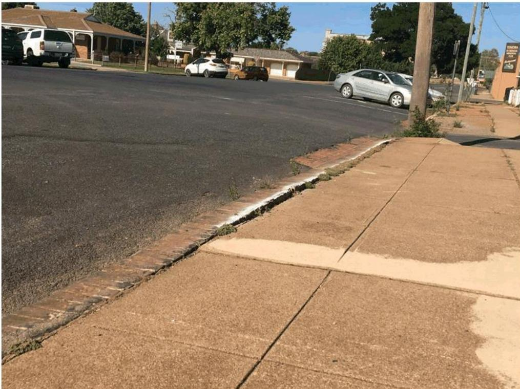
Photo 6 – Kerb and footpath defect
