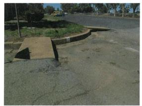
Photo 2; Example of substandard pedestrian gutter crossing bridges
