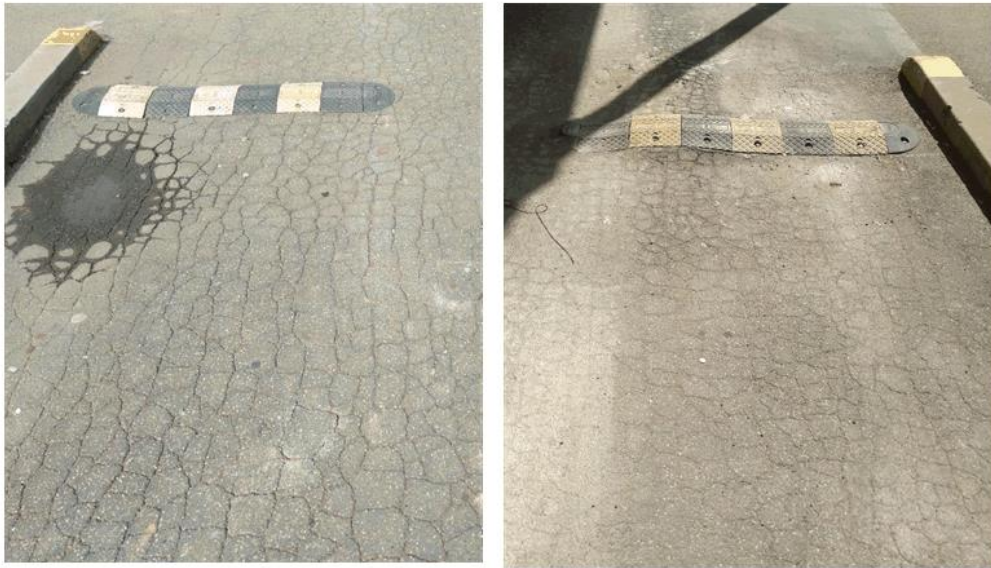
Image 3 & 4: Close up views of failing pavement with some gravel fines observed coming through the asphalt surface
