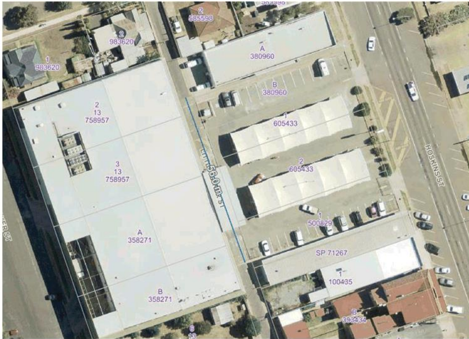
Image 1: Aerial overview of Little Baker St Asphalt Pavement
