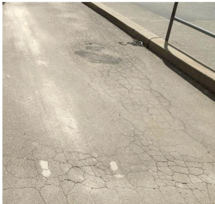
Image 5: Pothole failure that has received previous maintenance patching
