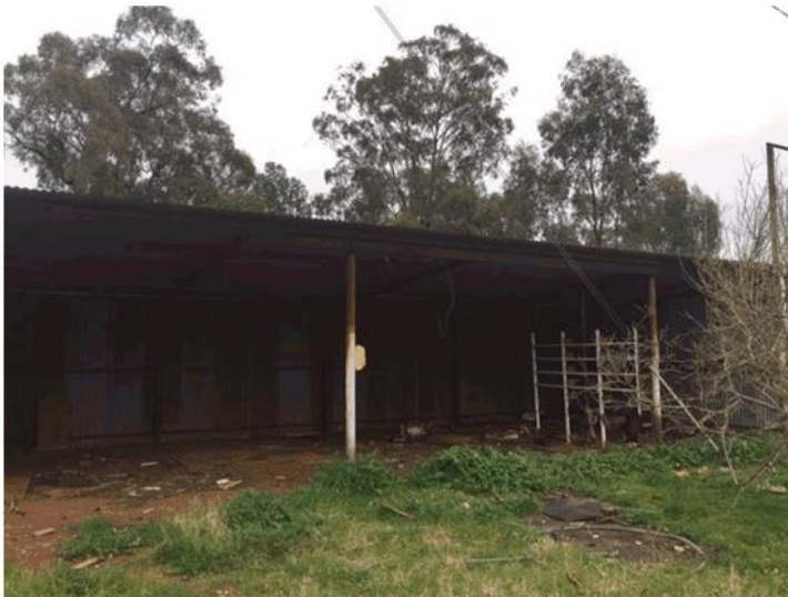
Photo 2: Shed located on Lot 1112
