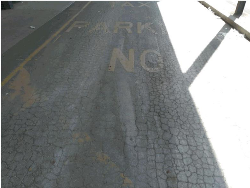
Image 6: Close up photo of failing pavement condition adjacent to entrance doors to Woolworths
