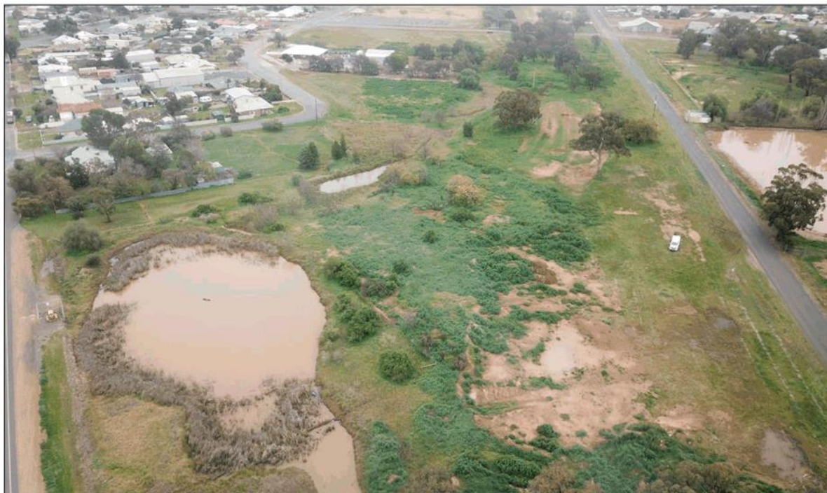
Existing dam 2 on site and adjacent lands plus dam 1 on opposite side of Gardner Street
