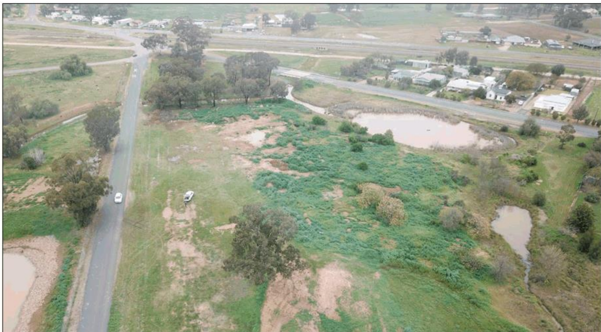
Image looking south over existing stormwater structure and lands for proposed dam
