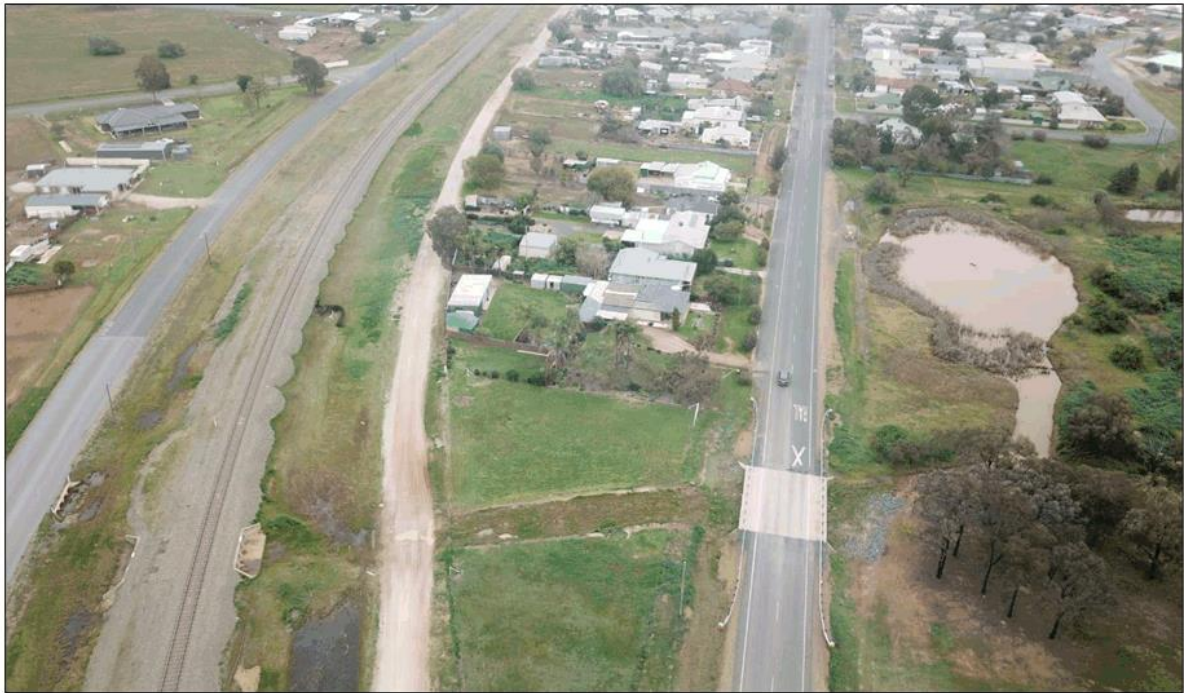
Existing dam 2 and downstream release to drainage lines releasing through railway lands
