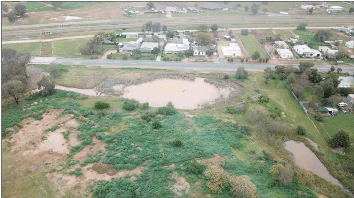
Image looking over existing stormwater structure and toward SW Note – the natural flow line from bottom right of photo and release to left.
