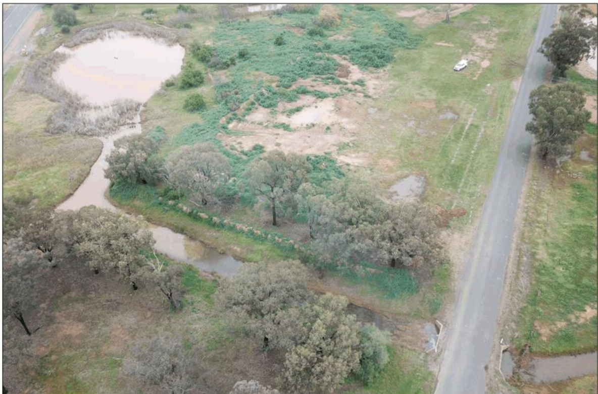
Dam 2 release and other catchment flow lines below proposed structure currently
