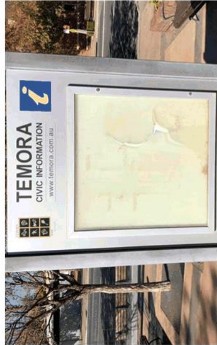
Info sign: Cracked Perspex (Paleface Park)
