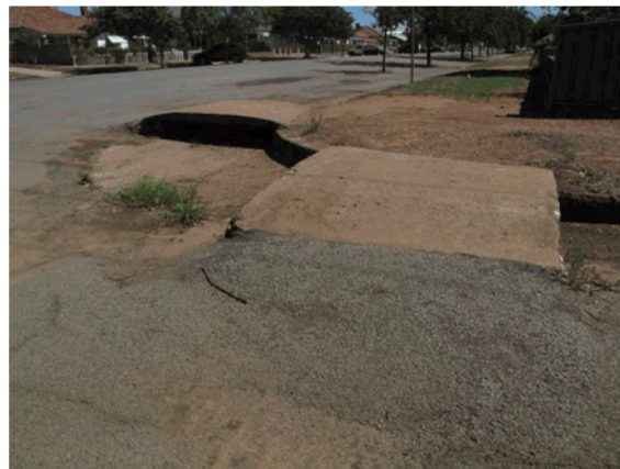
Photo 1; Example of substandard pedestrian gutter crossing bridges
