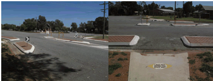
Photo's: Pitt Street, Ariah Park – Pedestrian Refuge Island and Blisters (Project completed in 2018)
