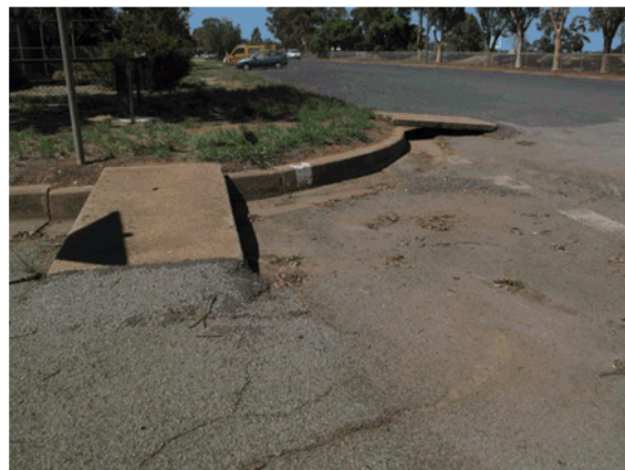
Photo 2; Example of substandard pedestrian gutter crossing bridges
