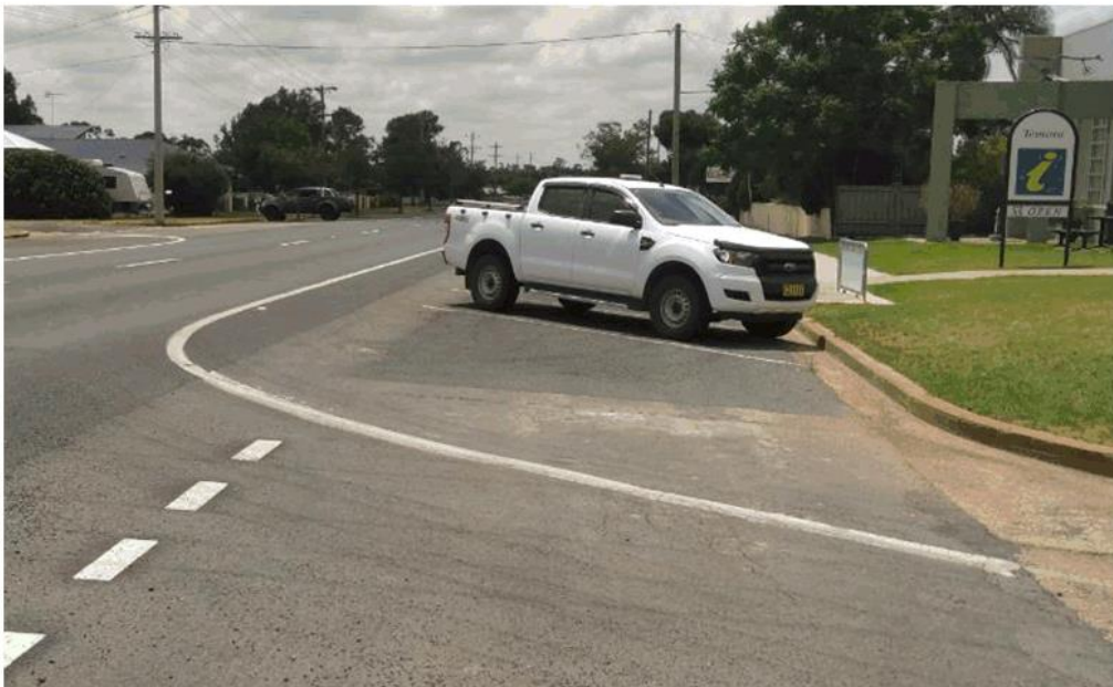
Image 2: Impeded sight distance looking right turning out of Macauley Street
