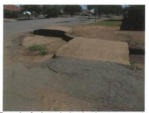
Photo 1; Example of substandard pedestrian gutter crossing bridges
