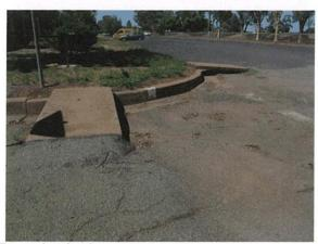
Photo 2; Example of substandard pedestrian gutter crossing bridges
