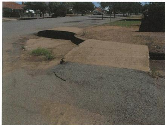
Photo 1; Example of substandard pedestrian gutter crossing bridges
