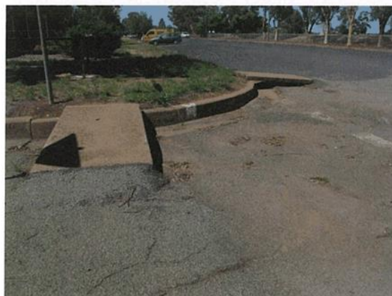
Photo 2; Example of substandard pedestrian gutter crossing bridges
