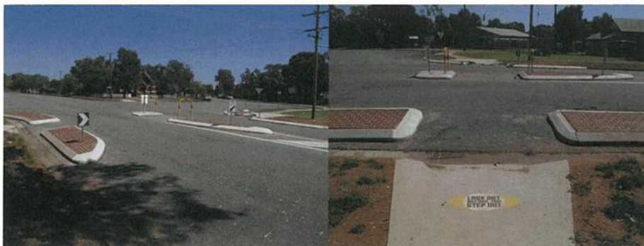
Photo's: Pitt Street, Aria Park – Pedestrian Refuge Island and Blisters (Project completed in 2018)
