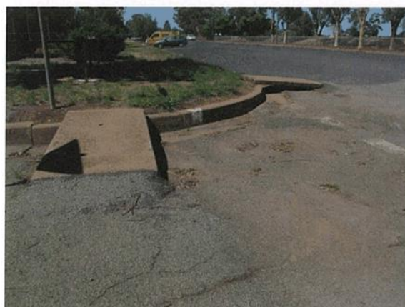
Photo 2; Example of substandard pedestrian gutter crossing bridges
