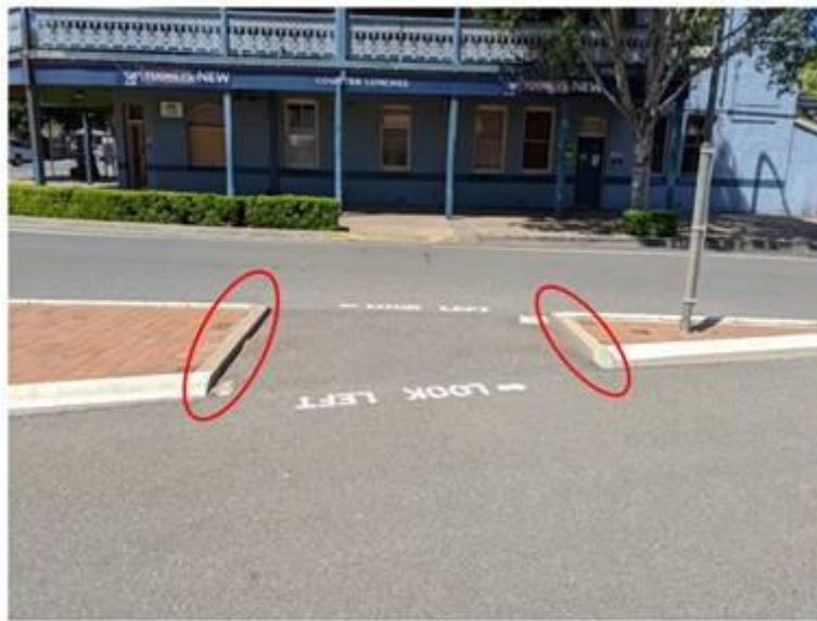
Attachment 2: Concrete edging example
