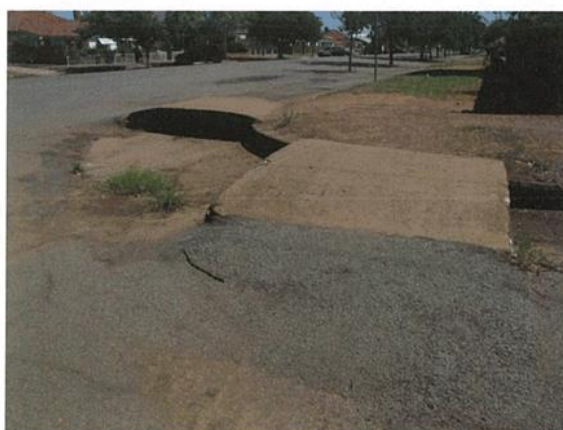
Photo 1; Example of substandard pedestrian gutter crossing bridges
