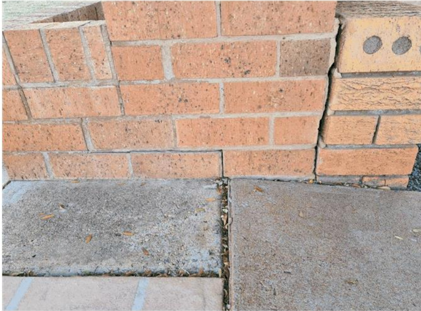
Image 1: Cracking to mailbox and fence
