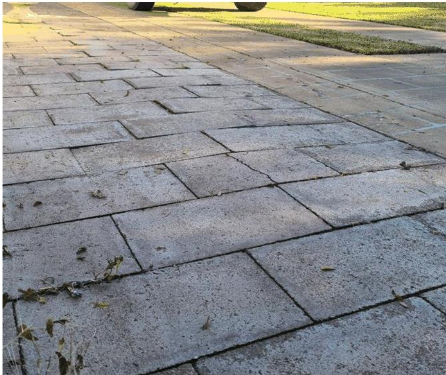
Image 4: Lifting row of pavers alongside driveway causing water ponding
