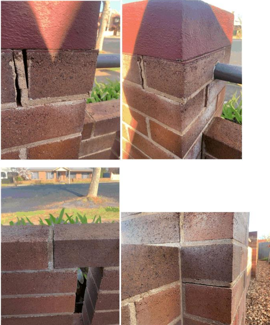
Image 6, 7, 8 & 9: Property Fence Damage starting to occur
