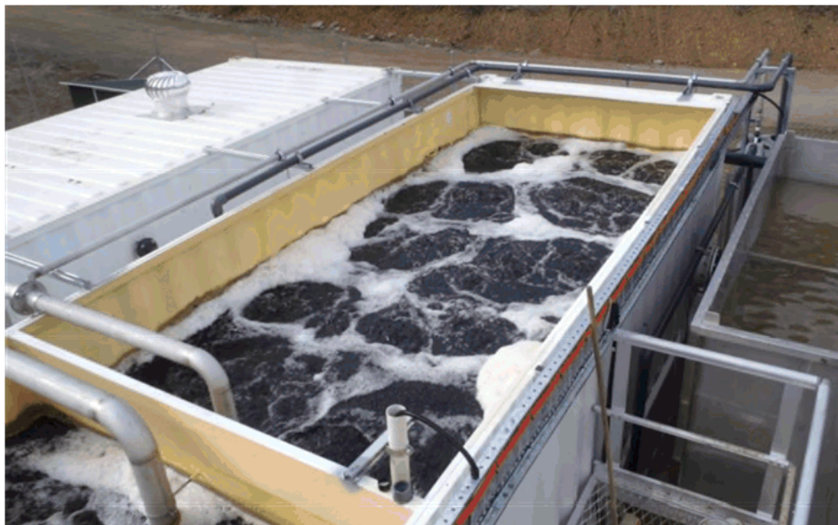
Figure 2-5: Package IDEA tank at John Moroney Correctional Centre
