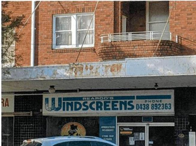
Rusted rods, fascias and soffit
