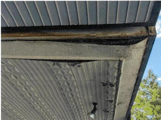
Rust damage and insecure soffit lining
