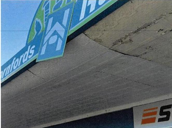
Water damaged loose soffit
