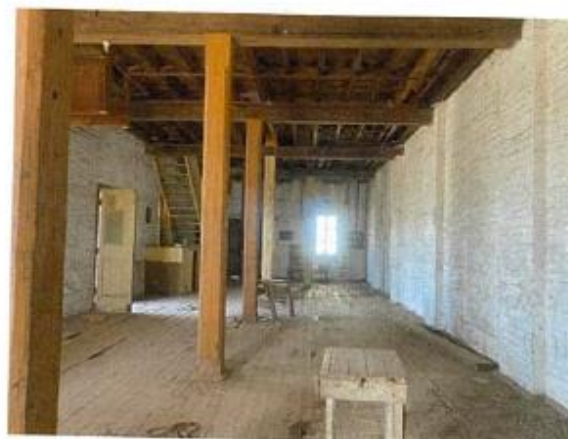
Plate 3.4: The eastern side of the ground floor looking south. The floor is severely compromised by termite damage. (18 November 2021)
