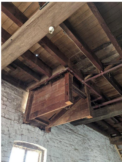
10. Internal view of the delivery chute, to be cleaned and retained in-situ.
