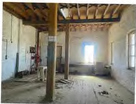
Plate 3.3: Interior of the eastern side of the ground floor looking north. The floor is severely compromised by termite damage. (18 November 2021)
