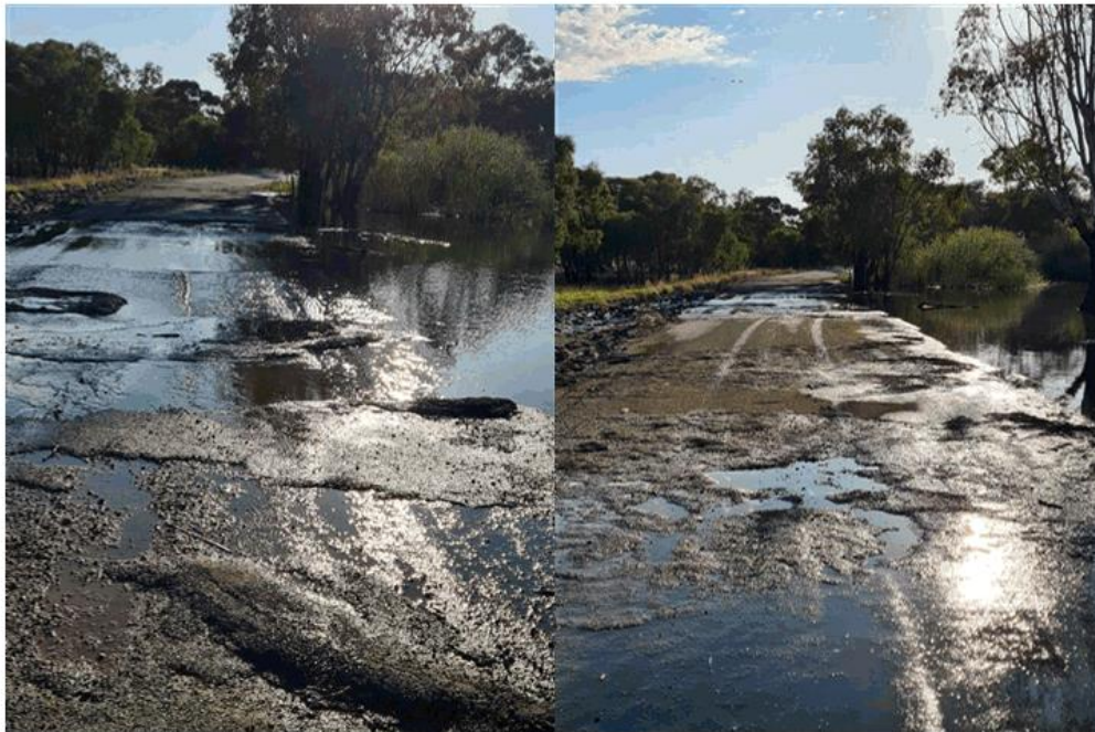
Images 4, 5 & 6: Bitumen Seal peeled of Lake Centenary Spillway following restoration works due to heavy rainfall in March 2023 which saw the Airport record 113mm in 4 hrs
