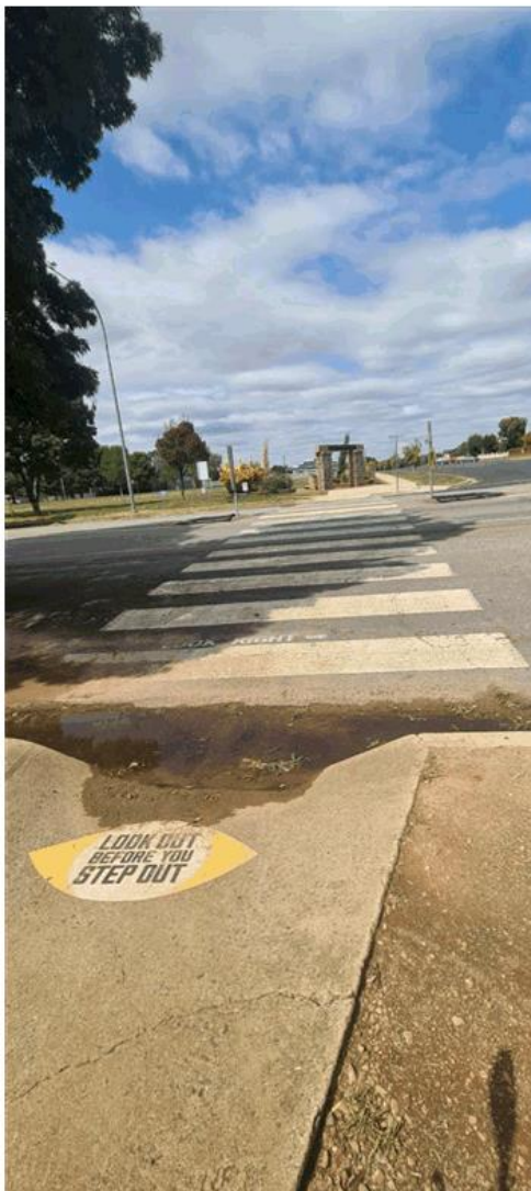
Image 1: Provided by resident with correspondence showing water ponding at pedestrian kerb ramp
