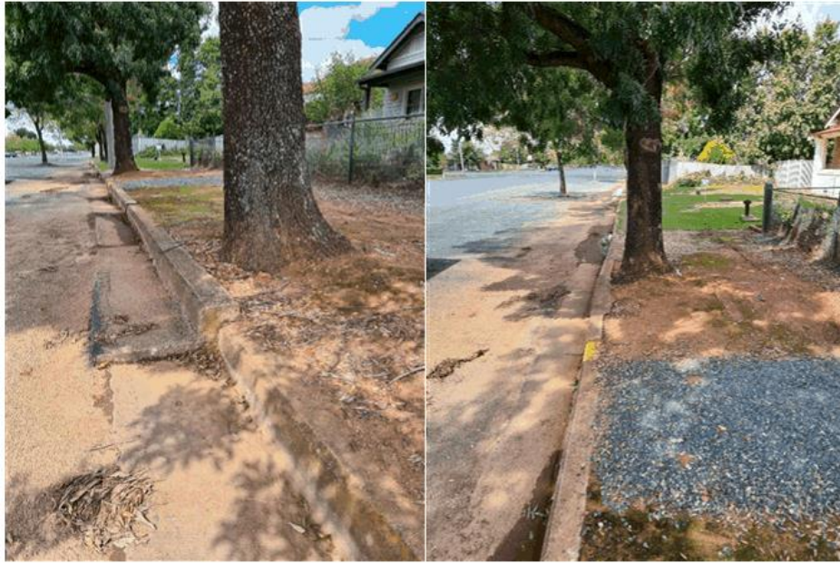
Image 4 & 5: Trees on nature strip outside 82 and 84 Crowley Street lifting the kerb and pushing the kerb out towards the road
