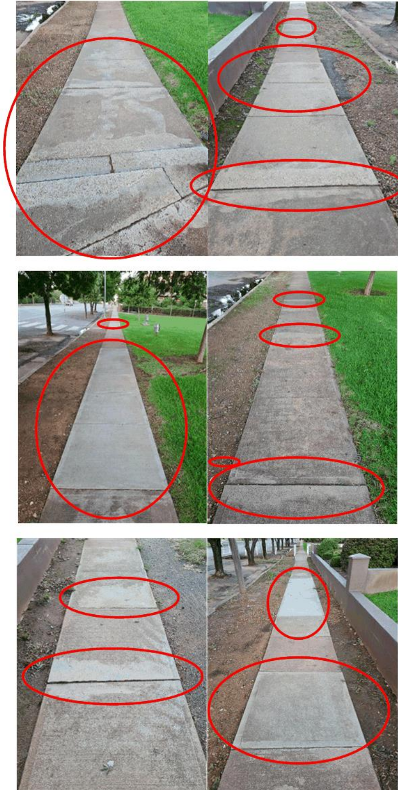
Images 10, 11, 12, 13, 14 & 15: Damaged concrete footpath along Loftus Street due to tree roots (Sections replaced or grinded indicated on images)
