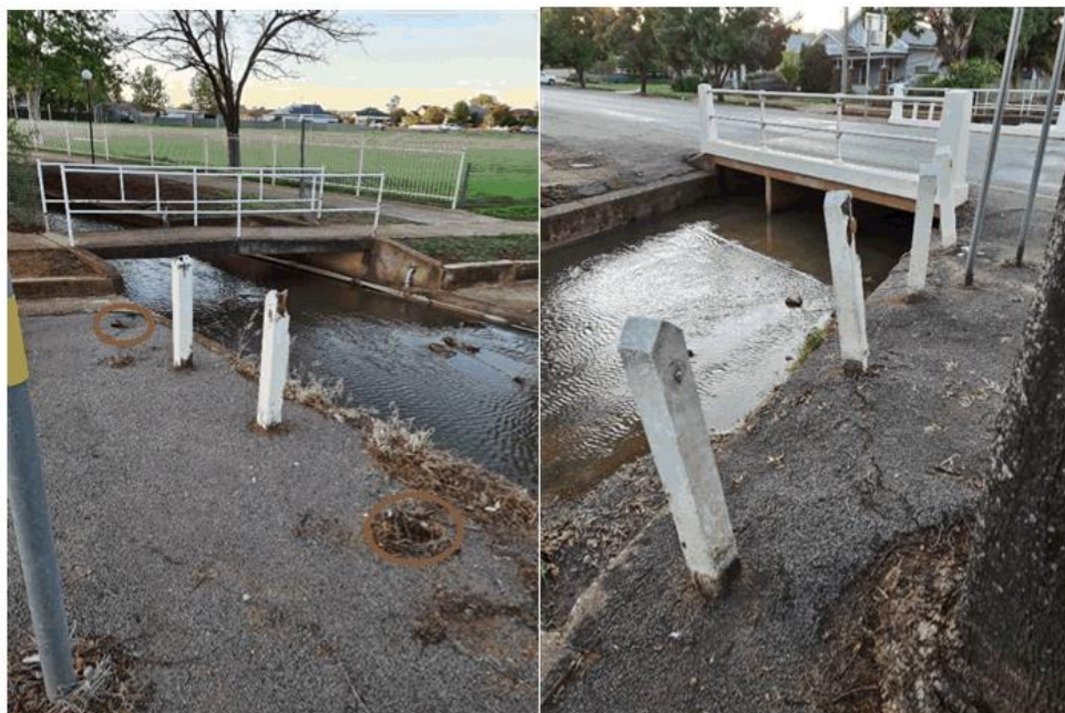
Images 20 & 21: Old timber bollards both sides of Loftus Street stopping people driving into the open drain need replacing as they are rotting and on Southern side 2 out of 4 are missing.
