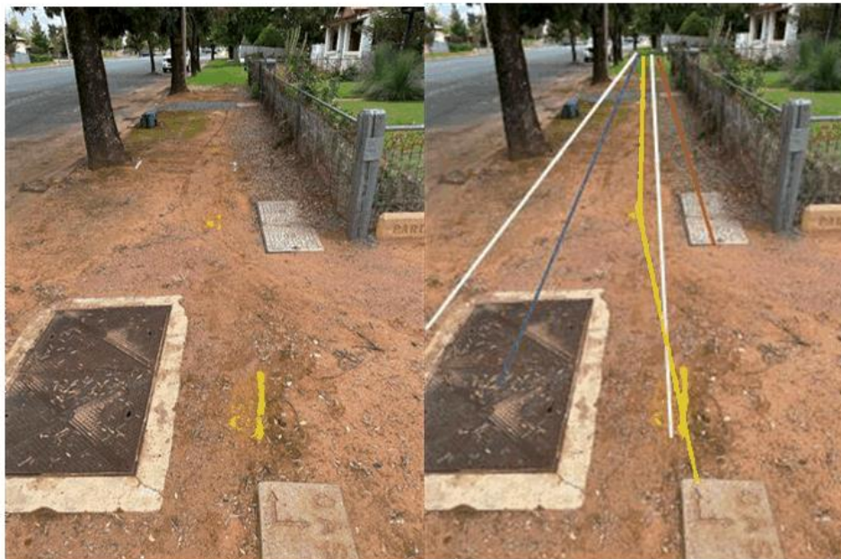
Image 6 & 7: Path Alignment along Crowley Street with Services marked on Image 7. Path offset 1m from property boundaries allowing inside edge of path to end up between Gas Line and NBN line so when boxing the path pegs aren't driven into services.
