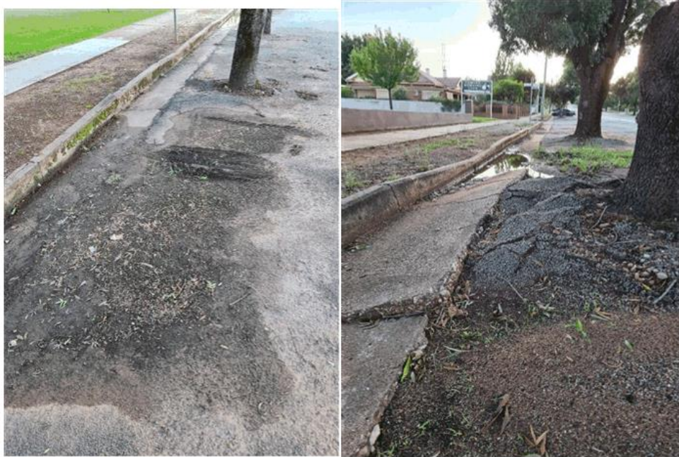
Images 6 & 7: Damaged kerb and gutter from tree roots along with dirt/mud settling from water ponding along with lifted road pavement
