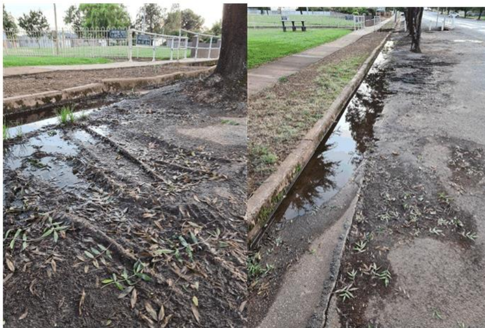
Images 4 & 5: Damaged kerb and gutter from tree roots along with dirt/mud settling from water ponding
