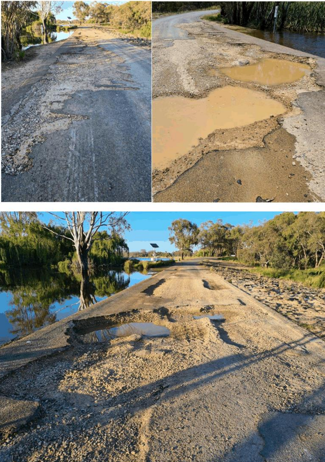
Images 1, 2 & 3: Flood damaged spillway at Lake Centenary following natural disasters in late 2022, prior to restoration works to stabilised and shape the pavement.
