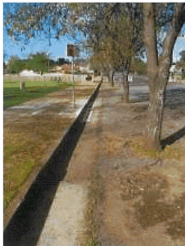
Image 1: Area showing lifting of pavement and high kerb.
