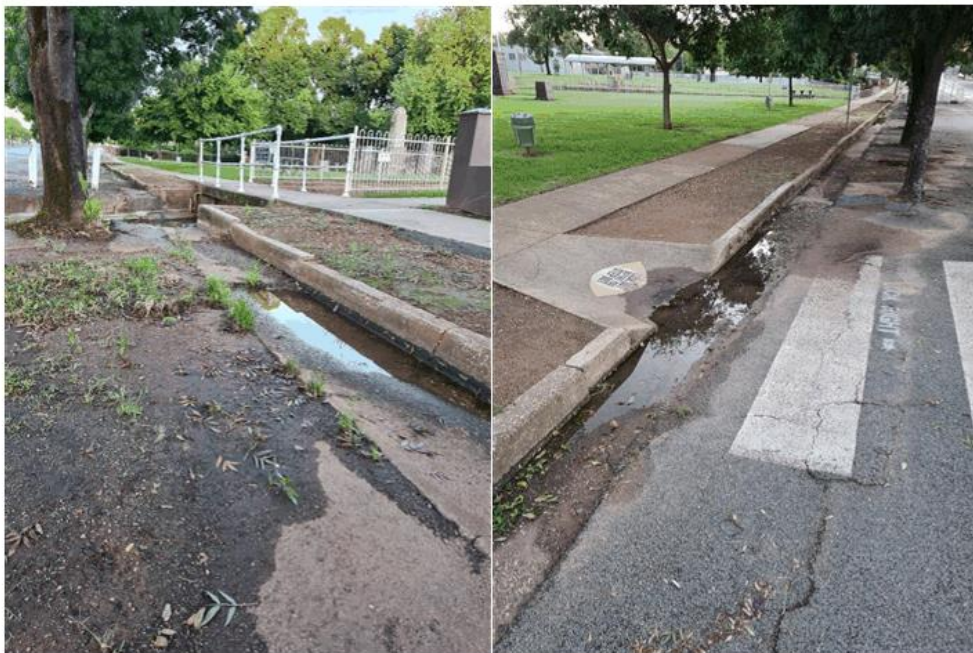
Images 8 & 9: Damaged kerb and gutter from tree roots along with dirt/mud settling from water ponding along with lifted road pavement
