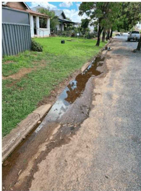
Image 3: Water ponding due to kerb movement and lifting from tree roots
