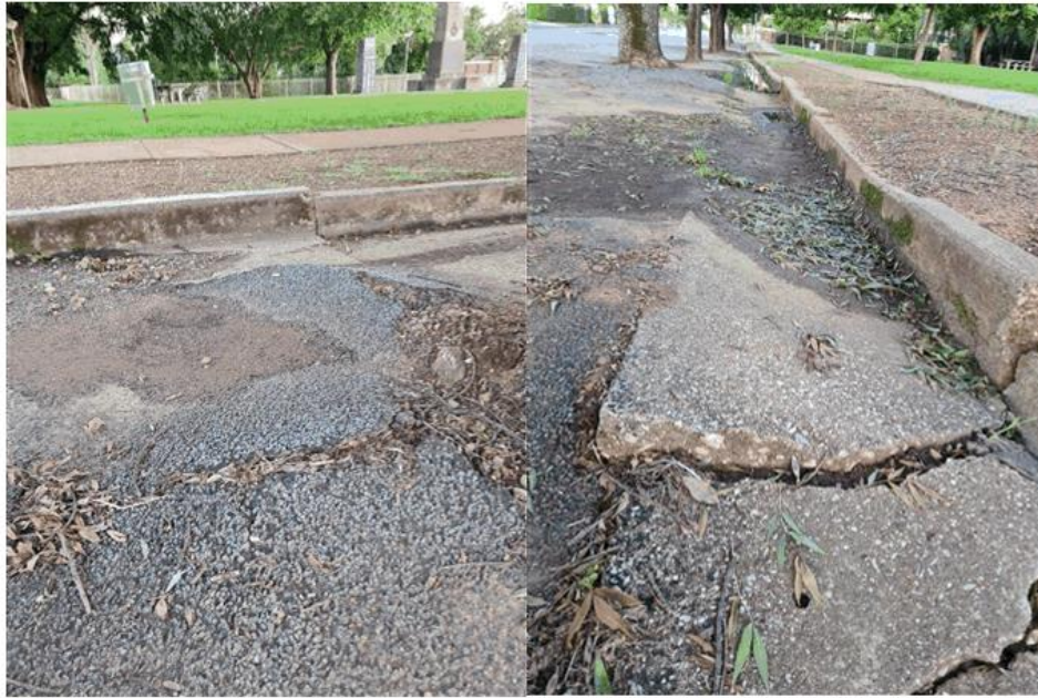
Image 2 & 3: Damaged kerb and gutter from tree roots along with lifted pavement
