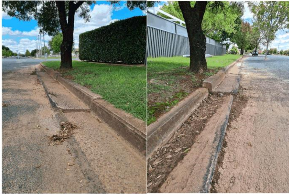
Images 1 & 2: Kerb lifting due to Ash tree alongside 75 Polaris Street (in Crowley Street)
