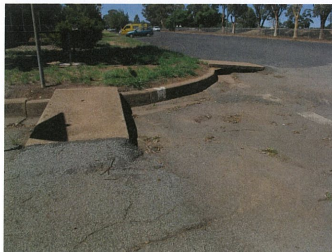
Photo 2; Example of substandard pedestrian gutter crossing bridges
