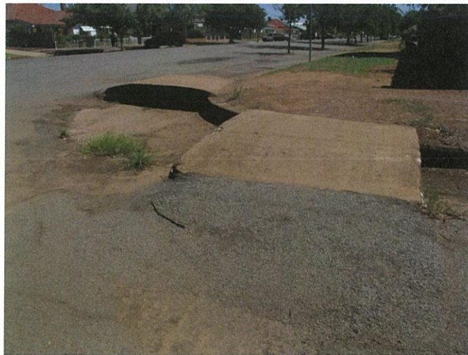
Photo 1; Example of substandard pedestrian gutter crossing bridges
