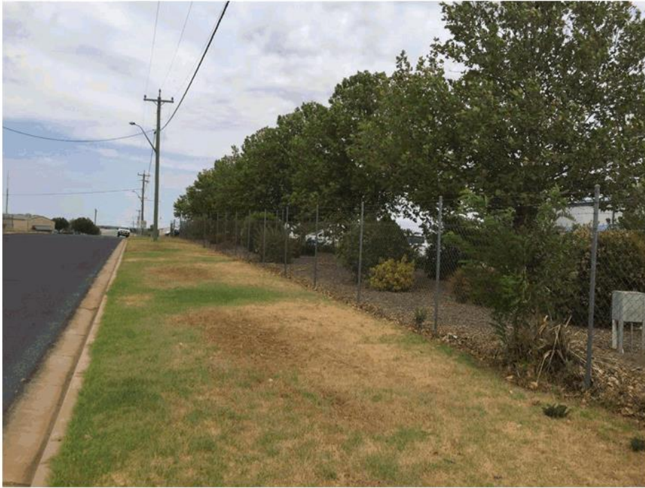
Photo 3: Hakea Street frontage
