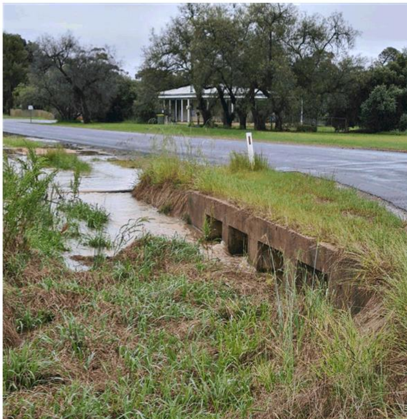
Culverts running under Murphy Street to the Railway Line
