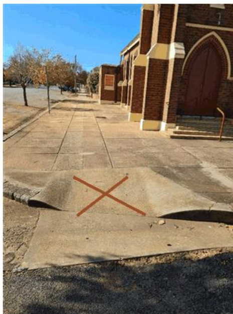
Image B: Remove existing kerb ramp on Eastern Side, reinstate kerb and gutter plus footpath behind
