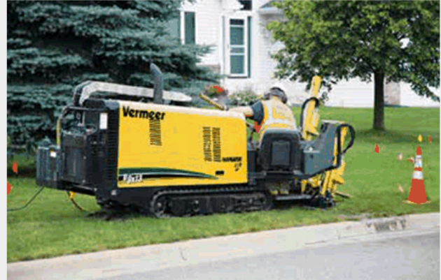
Trenchless - Horizontal Directional Drilling
