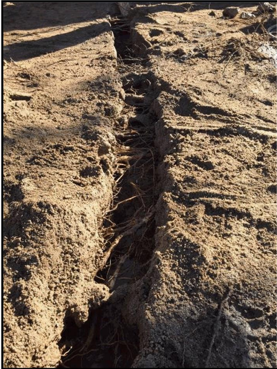
Figure 2 – The open trench showing exposed tree roots.
