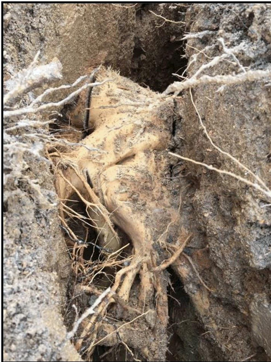
Figure 3 – An example of some of the larger woody tree roots exposed, and then cut cleanly.
