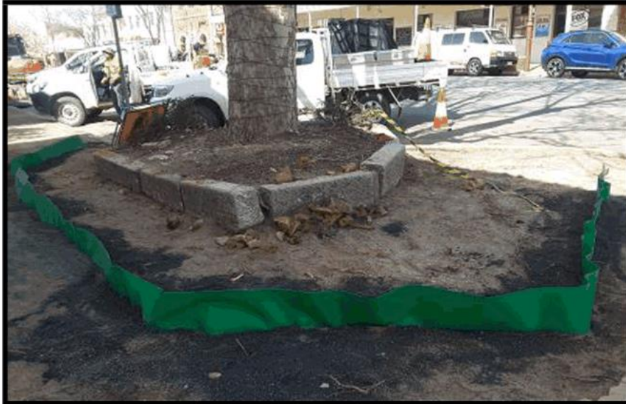
Figure 4 – Root barrier material installed and trench backfilled, prior to (new) paving being laid on the tree's surrounds.
