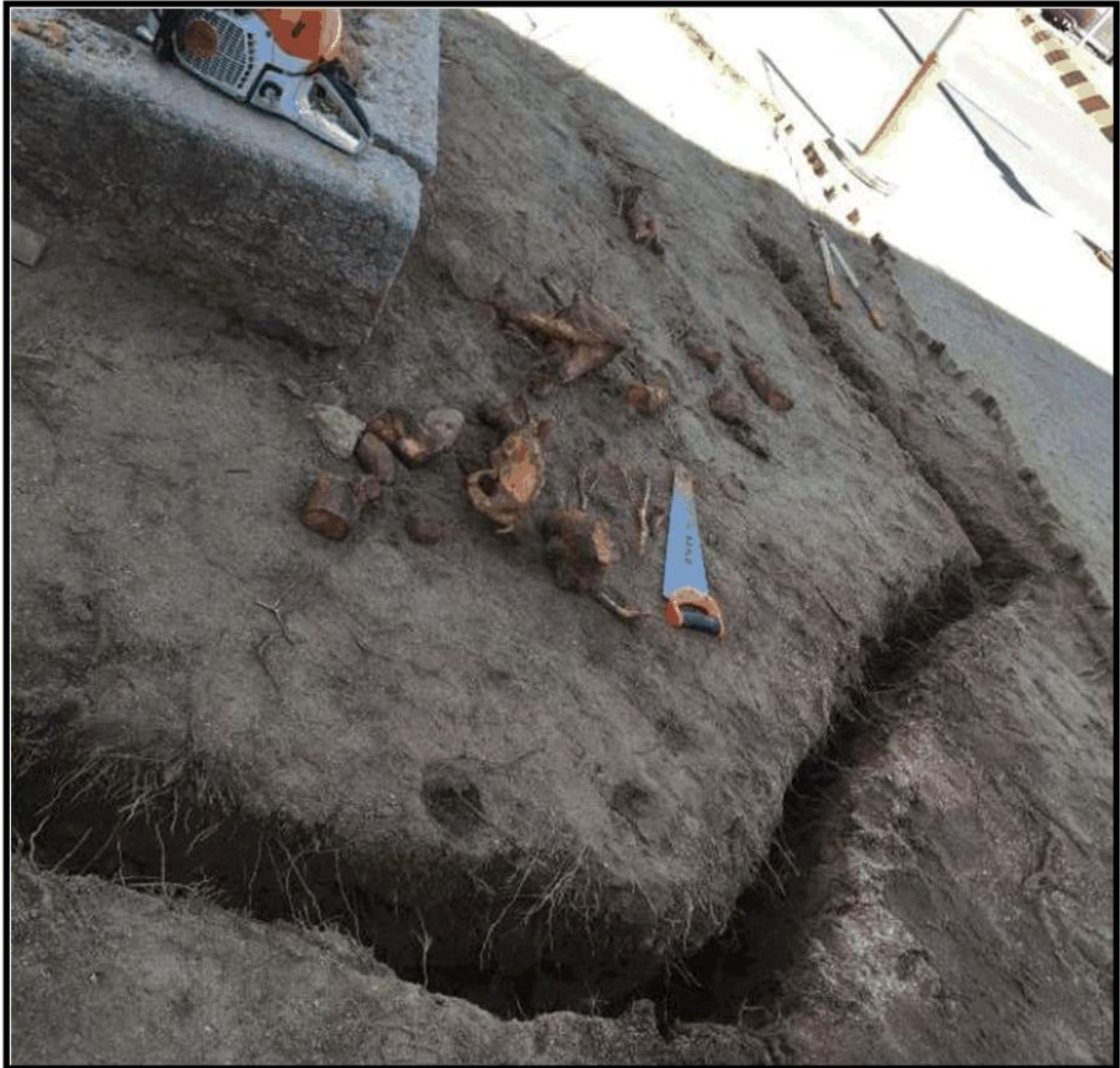
Figure 4 – Root pruning completed with the range of “root segments” removed from the trench laid out.
