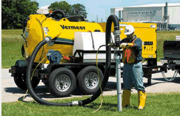
Hydro Suction Footing Excavation
