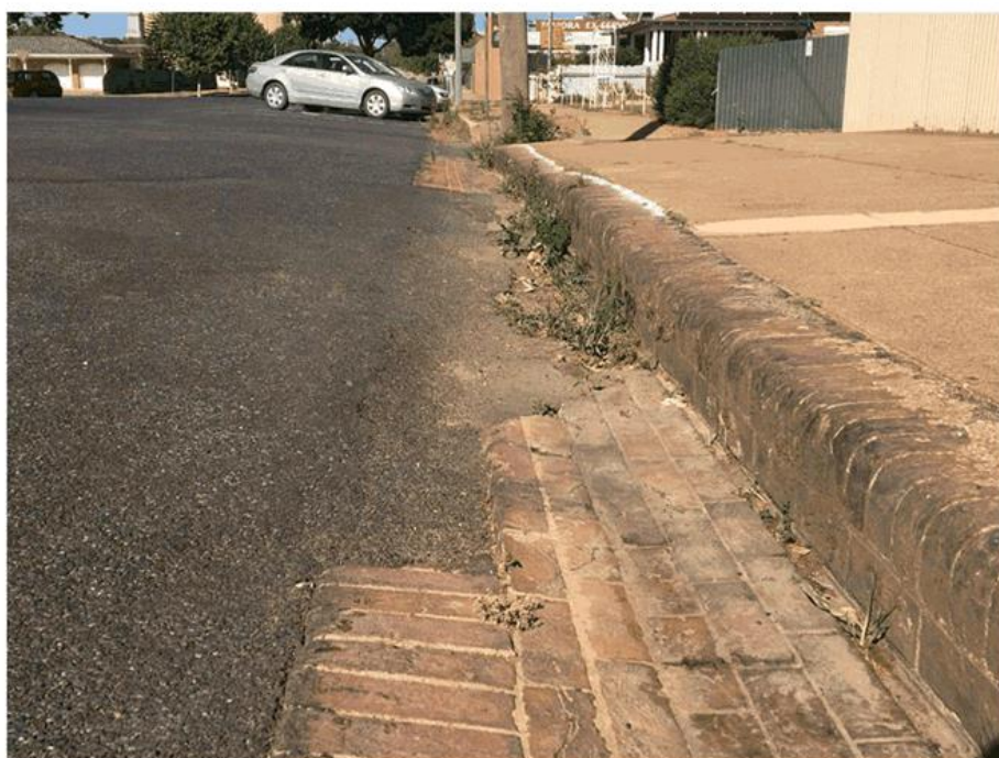
Photo 5 – Kerb defect
