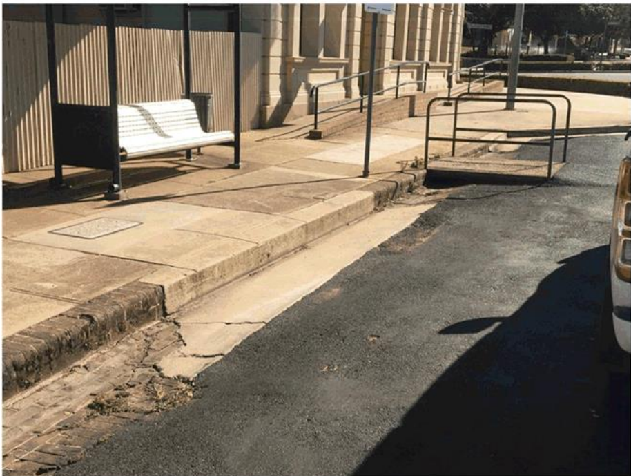
Photo 4 – Kerb defect
