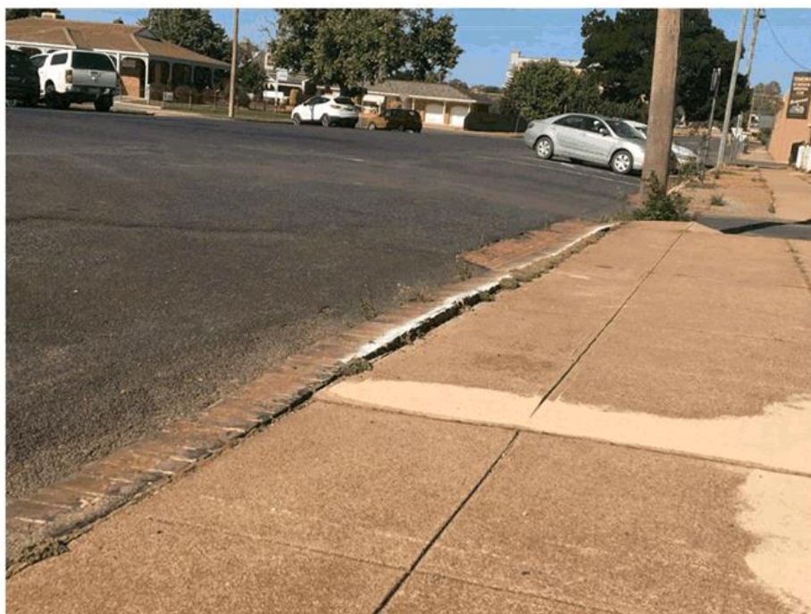
Photo 6 – Kerb and footpath defect
