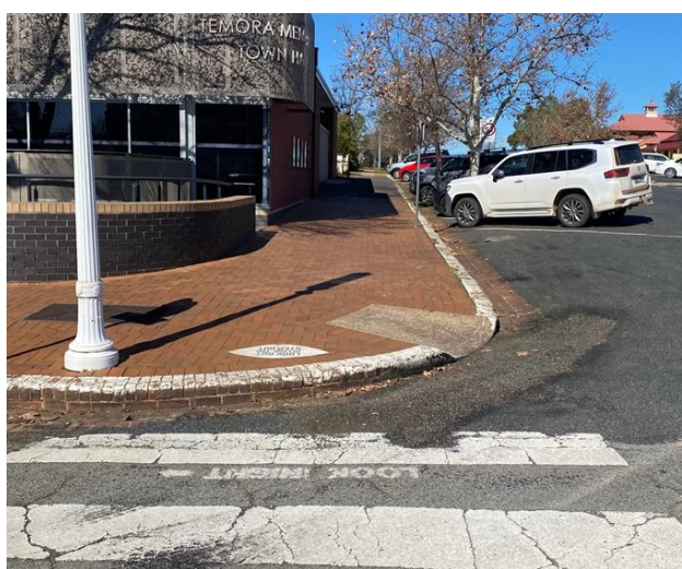
Kerb adjacent to St Annes School
