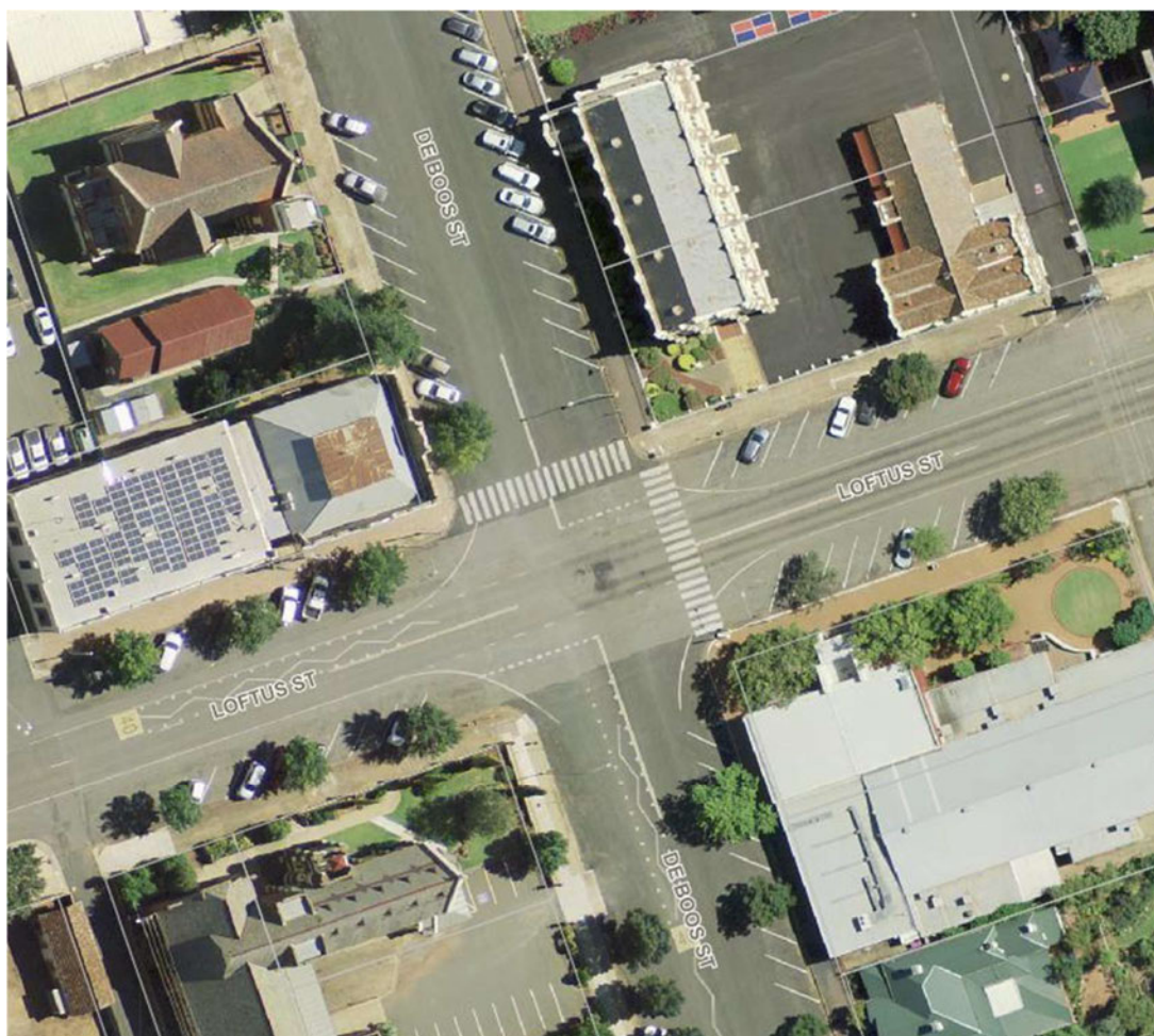
Figure 5: Current De Boos Street/Loftus Street intersection
