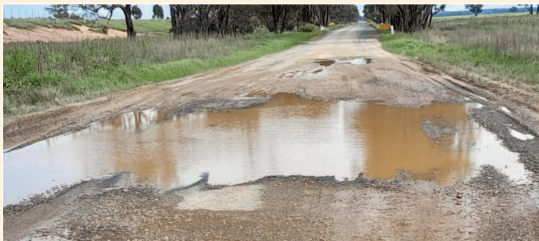
Pictured is the damaged bitumen causeway on Howards Road. The road has been closed since early August and this image shows the significant damage caused by recent weather events. Council has not yet been able to determine a date to undertake restoration works on this road.
